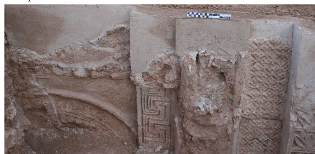
Figure 11. Delineation of the boundary between the protective plaster layer and the original stucco surface achieved through the recession and texturing of the protective render
