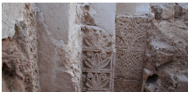
Figure 11. Delineation of the boundary between the protective plaster layer and the original stucco surface achieved through the recession and texturing of the protective render
